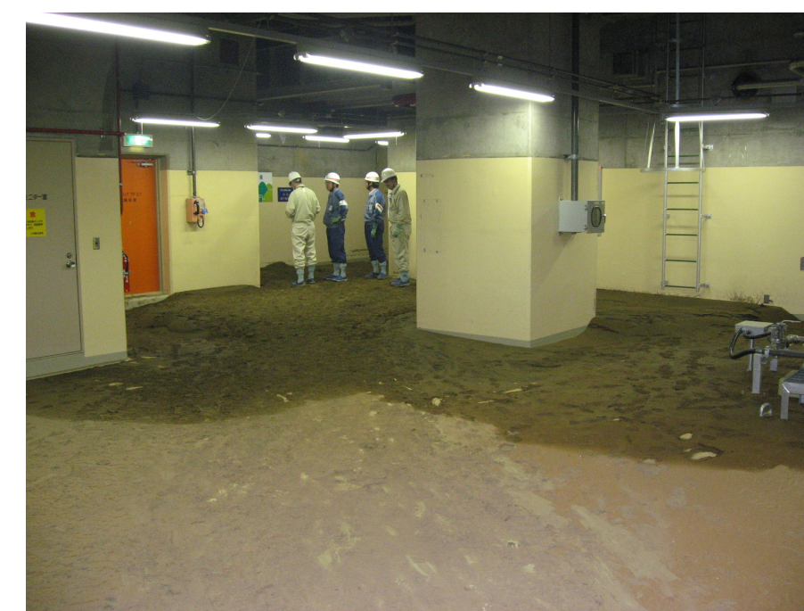
Mud accumulated on the floor under the inflow hole
